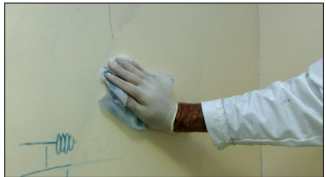
Graffiti removal in progress
