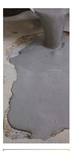
"It doesn't take long for a concrete floor with minor damage to deteriorate. The worse it gets, the more costly the repairs and the more downtime needed. With Watco Flowpatch you can fix floors fast – it's our quickest and easiest to use repair mortar and can be used anywhere by anyone."
